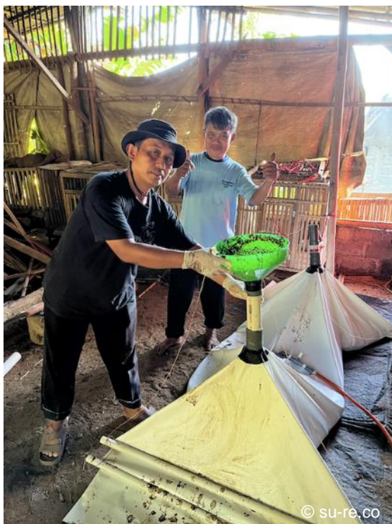
Top-load biogas digester in Gunung Kidul managed by Pak Rubani and Pak Mugi.
